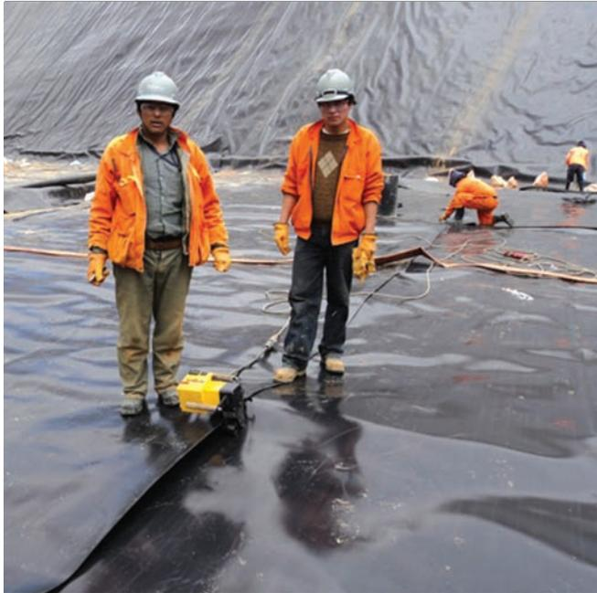
El Aliso workers installing liner materials at Yanacocha.
