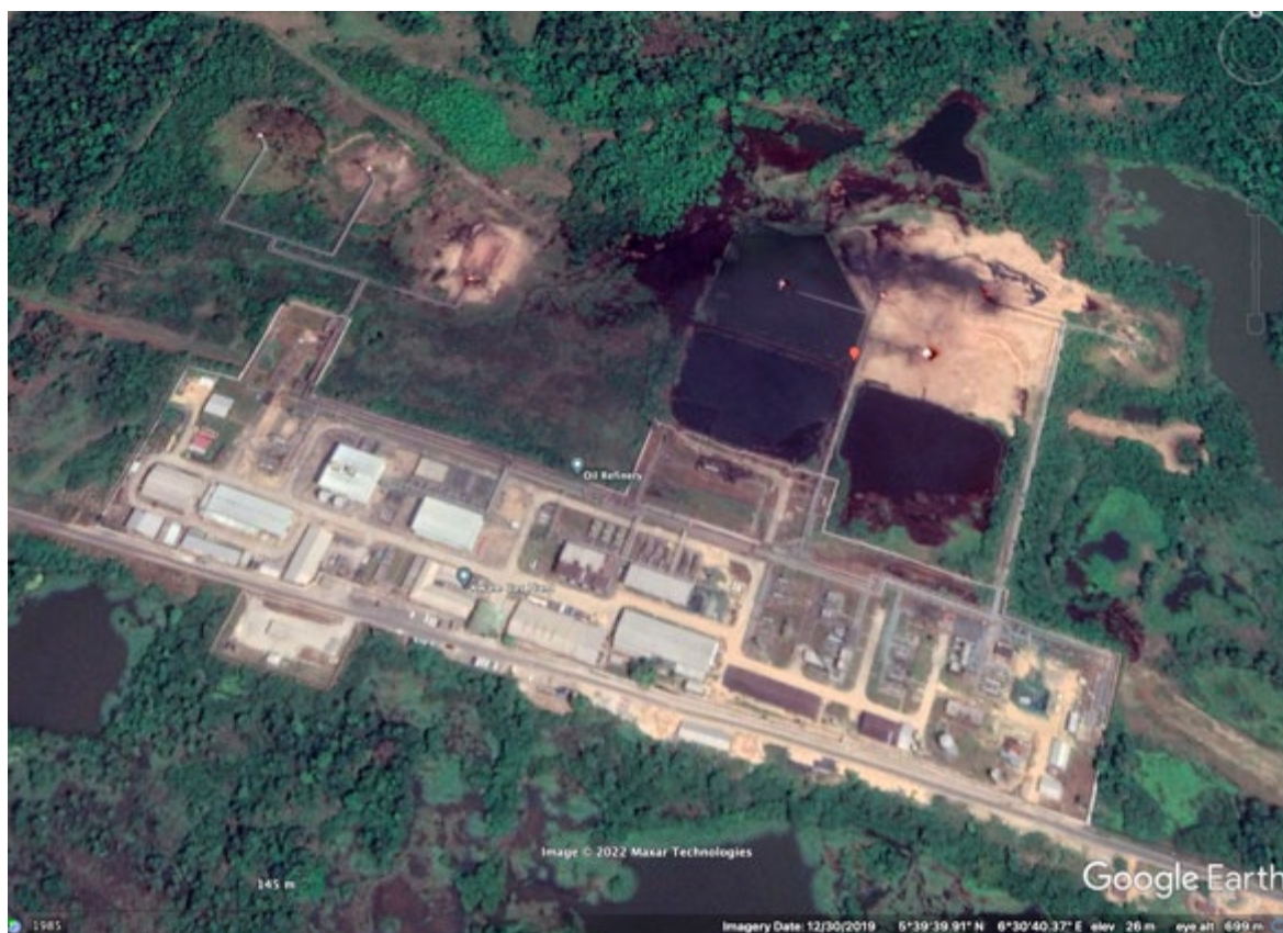
Figure 26: Kwale gas plant with gas flares
