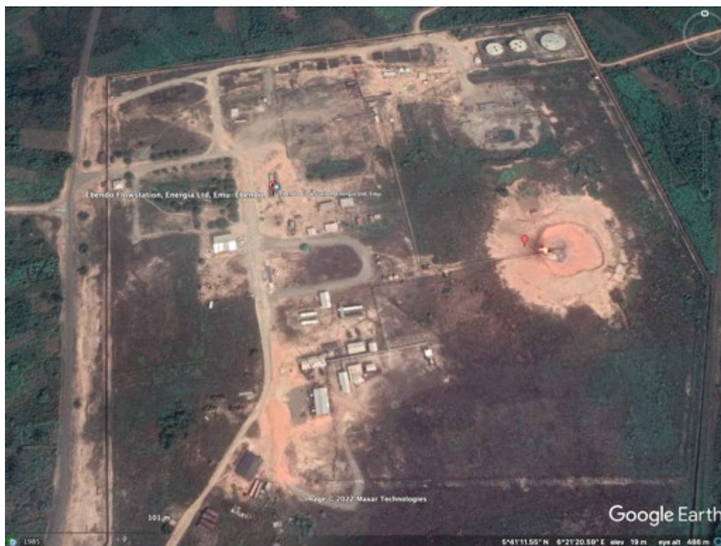
Figure 44: Detail of the Ebendo plant
