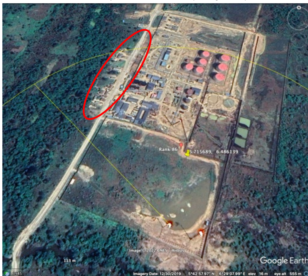
Figure 22a: detail of the location of the super-emitter flare at Kwale (Sterling Beneku) flow station
