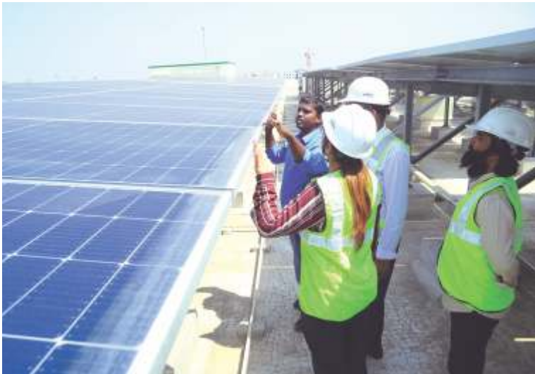
Figure 26: OPM team inspecting DMART plant
