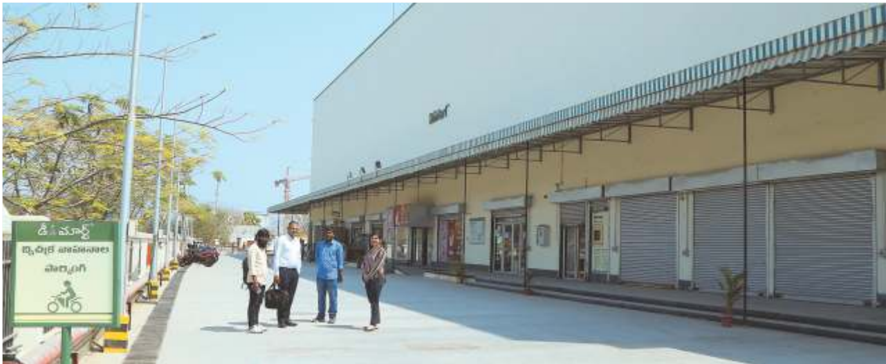
Figure 24: DMART complex in Hyderabad, end beneficiary for 4PEL
