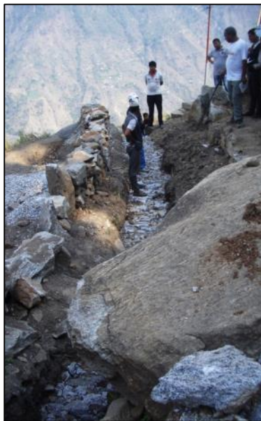
Photo 12: New branch canal (partially complete)
