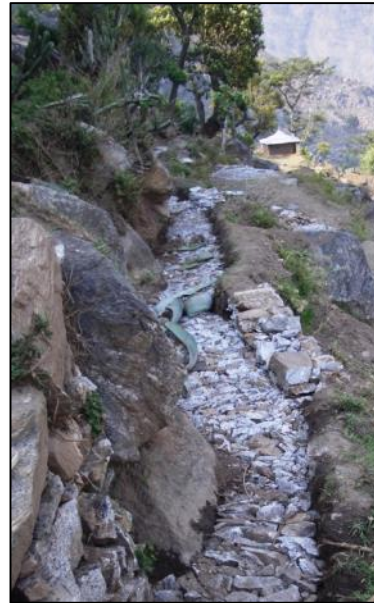
Photo 12: New branch canal (partially complete)
