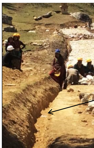
Photo 3: Side drain alignment
