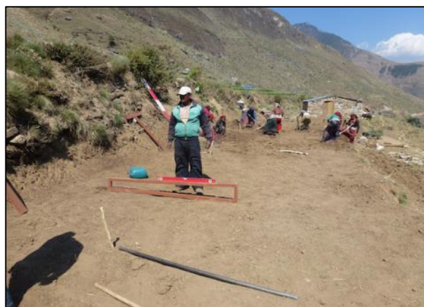
Photo 14: Use of camber template during training
